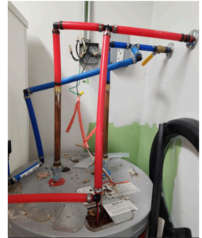
Obstructed electrical service equipment
