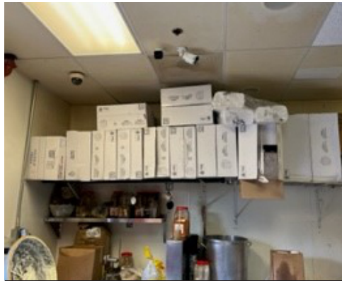
Improper storage of combustible materials
